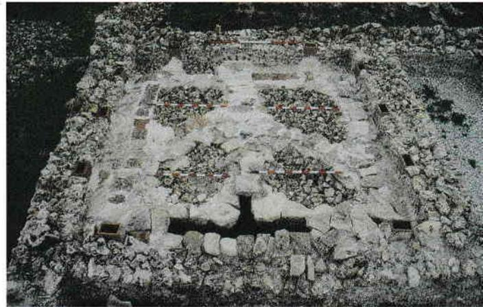
Fig. 4. Hypocaust room with the channels corbelled over and ready for the opus signinum floor to be laid. Photo: Peter Reynolds.
