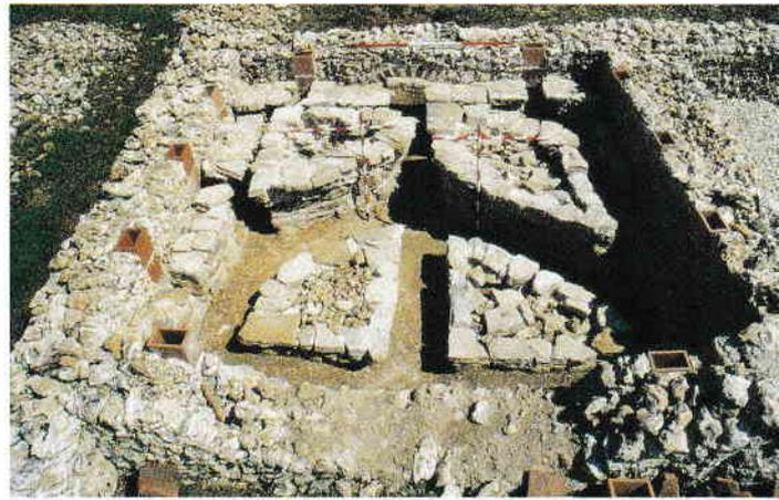
Fig. 3. Hypocaust room during construction showing the islands of Purbeck limestone, the channels and the tubuli in the walls and the praefurnian arch and stoke hole. Photo: Peter Reynolds.
